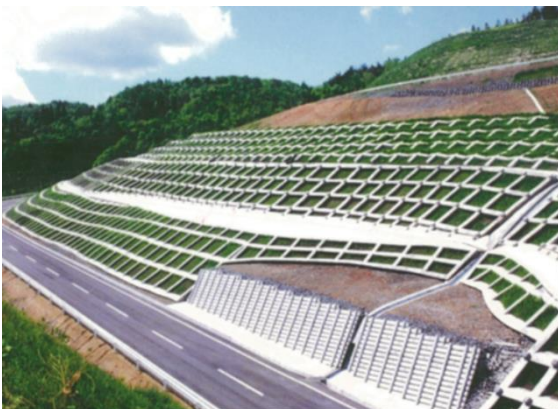
Slope stabilization
